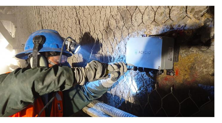
A major mining company in Peru wanted to measure displacement in the tunnel where its mineral conveyor belt is located. The company needed reliable readings of rock movement every six hours from the length of the approximately two-kilometre tunnel. The monitoring was complicated by potential signal interference from radio noise, magnetic fields, metals, pipes and other mine obstructions.
