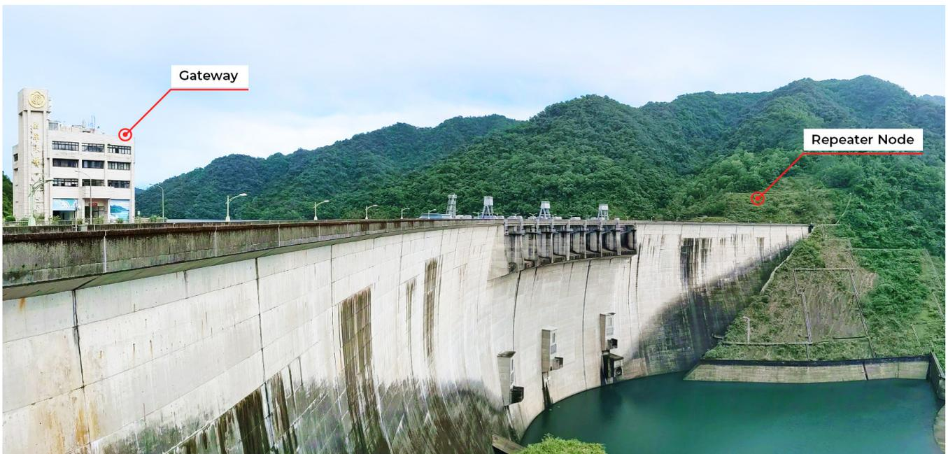
The nodes transmit readings to the Ackcio Gateway (BEAM-GW), installed on the top of the building on the dam that has WiFi and power. The system started reliably sending automated readings in October, a promising start to a two-year pilot project to test this system at the Feitsui site.
