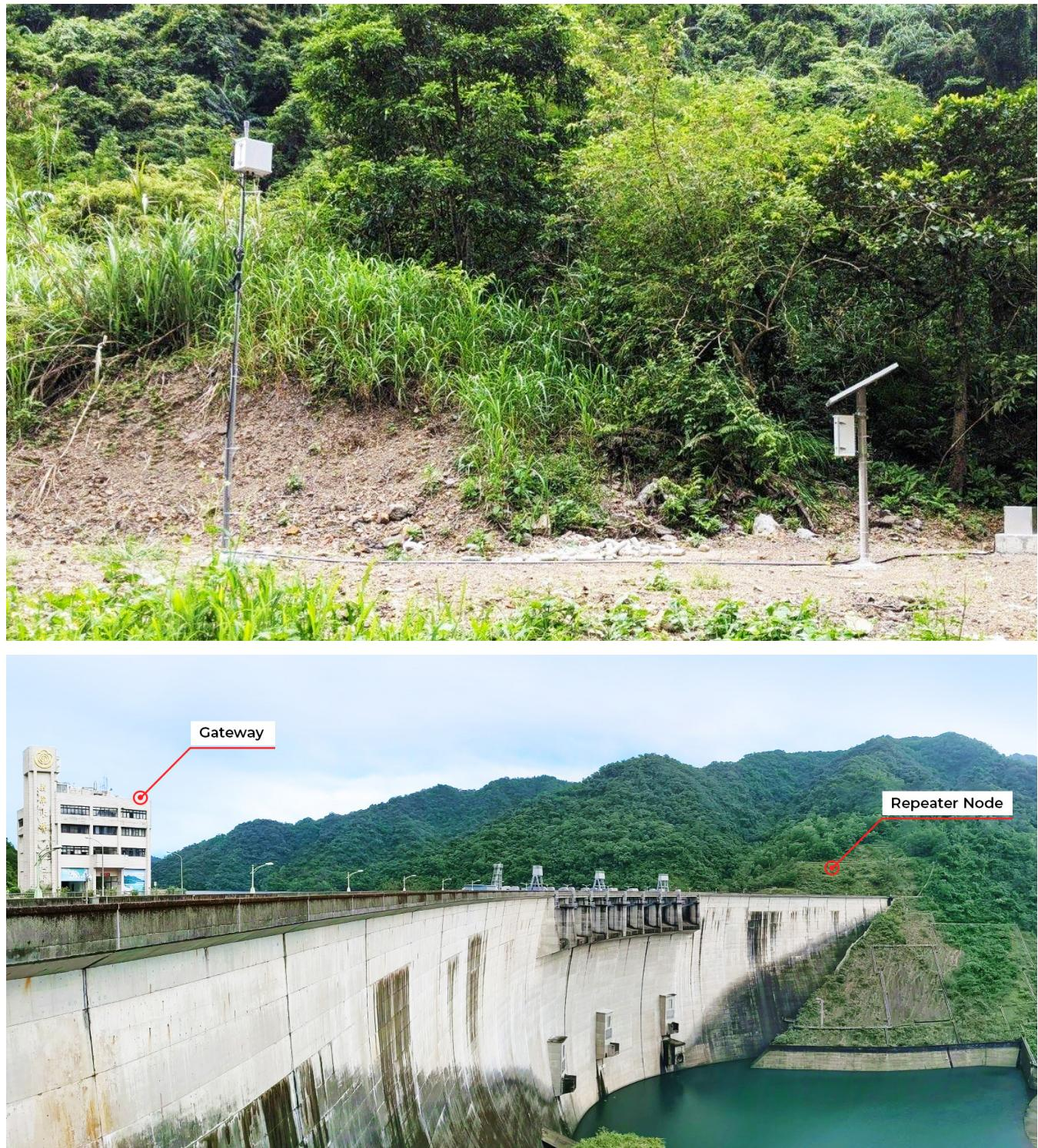
The nodes transmit readings to the Ackcio Gateway (BEAM-GW), installed on the top of the building on the dam that has WiFi and power. The system started reliably sending automated readings in October, a promising start to a two-year pilot project to test this system at the Feitsui site.
