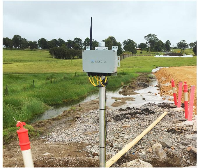
Tetra Tech Coffey chose the Ackcio Beam wireless data acquisition solution to monitor a preload over a soil section, where subsurface materials included up to 9 metres of soft, compressible estuarine sediments. The constructed embankment was approximately 700 metres long and up to 8 metres high.
