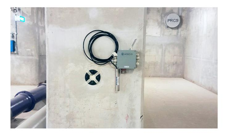
Soil Investigation chose the Ackcio Beam wireless data acquisition solution, as its unique mesh system allows for far deeper and longer data transmission, even in challenging underground conditions, where other wireless solutions based on LoRa or 2.4GHz mesh networks have reliability issues.
